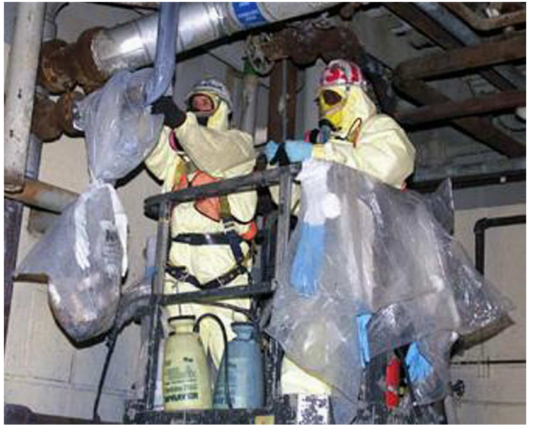
Workmen in appropriate safety gear remove harmful asbestos from a workplace
